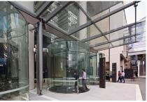
For International Towers 3 at Barangaroo, record Automatic Doors was responsible for a total of 7 revolving doors, including 4 of the largest Diamond Series doors ever built at 4000mm diameter x 3900mm high, installed to the South Lobby
