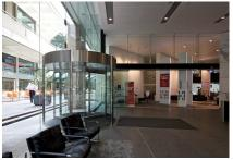
As part of the extensive ground floor building refurbishment to the plaza entry of NAB House, record Automatic Doors was engaged to provide a new revolving door entry. This required alteration works to the existing frameless glazing and a new automatic swing door entry, featuring the DFA 127 automatic swing door operator mounted under the slab to allow for a full frameless glass appearance.
