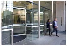
The lobby upgrade to One Farrer Place in Sydney involved replacing the existing 20 year old canopy style revolving doors with new fully frameless record Diamond Series revolving doors as preferred by the architects Johnson Pilton Walker.
