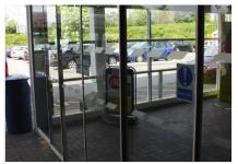
This is an installation of the **record uk** telescopic TSA20 at the Tesco store in Rugby. The store required an entrance capable of allowing the safe passage of large numbers of people at one time, and at the same time not leave the entrance open to the elements for unduly long periods. This was achieved by the installation of automatic folding doors at both sides of the wide entrance, thus allowing maximum access while mimimising rapid ingress of cold air and dicomfort for customers and staff.
